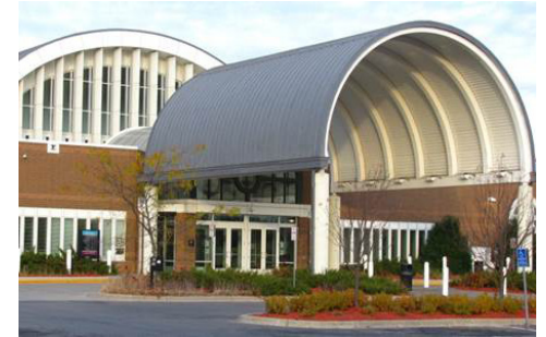
Vaulted roofs create visual interest
