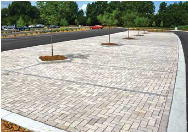
Pavers set within a concrete border divide a large asphalt parking area
