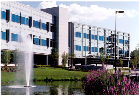
Building oriented to support views and daylighting while connecting to primary vehicular drop-off area
