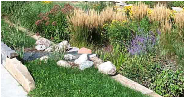
Parking lot run-off captured in a rain garden
