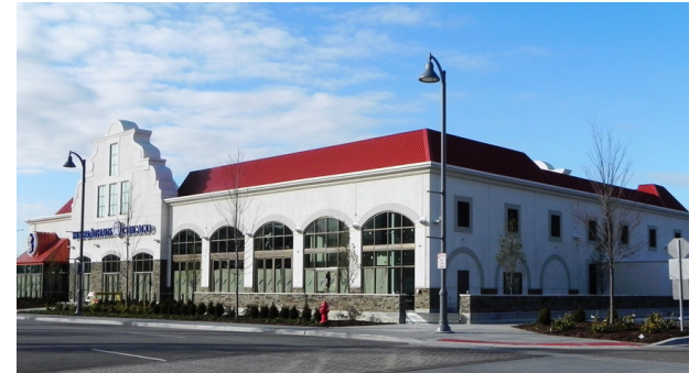
A false mansard roof, seen from the street, acts to screen rooftop mechanical equipment
