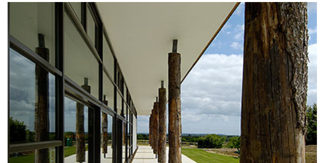
Reclaimed and recycled materials used in the design of a building
