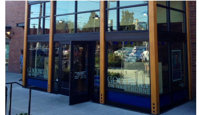
Aluminum storefront accented with wood creates a nice entry to a brick building
