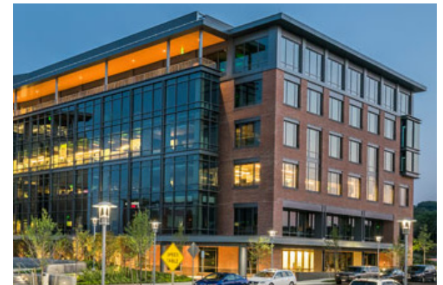
Punched window opening provide a contrast to the adjacent curtain wall
