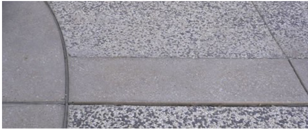
Smooth and exposed aggregate concrete provides visual interest
