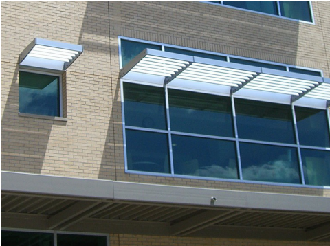
Proper orientation allows for solar gain in the winter and solar shading in the summer
