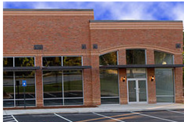
An arched clearstory breaks the repetitiveness of the facade and highlights the entry
