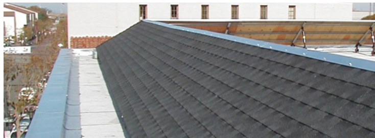
A false mansard roof, seen from above, acts to screen rooftop mechanical equipment
