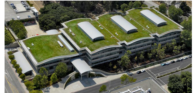
Green roofs can reduce stormwater runoff, energy use, and the heat island effect
