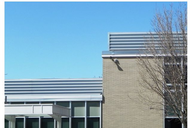
A short parapet of corrugated metal screens views of rooftop systems
