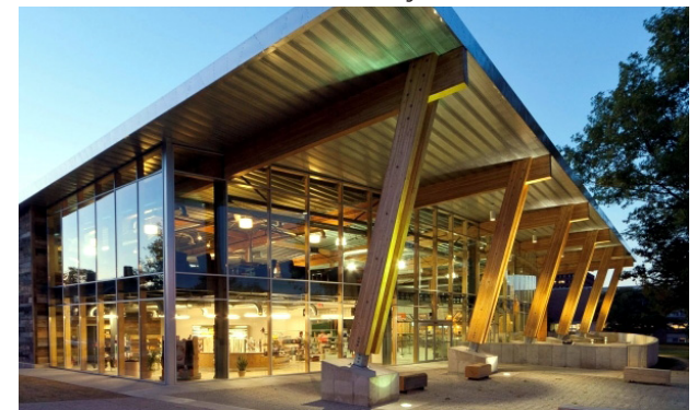
Large wood glulam columns and beams add warmth to a glass and aluminum facade
