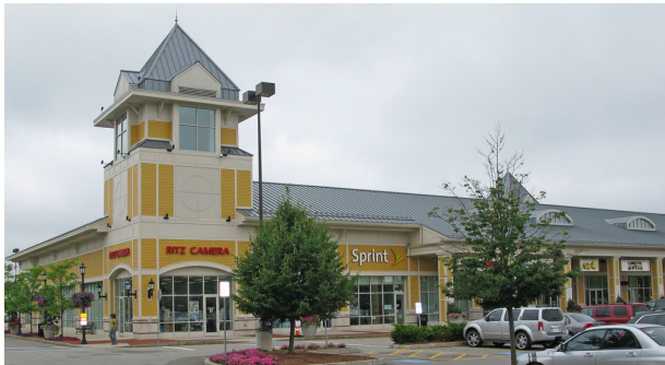
A highly detailed corner element anchors this well designed retail development
