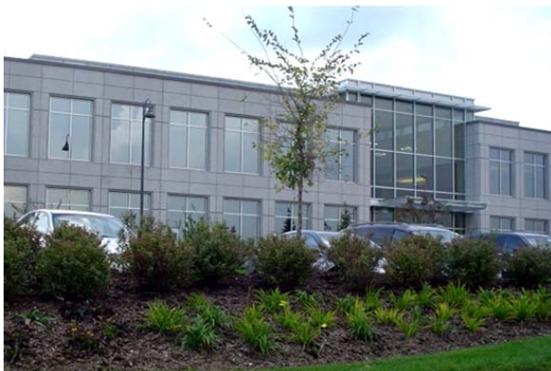
Screening of parking is achieved with a planted berm
