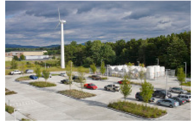
Parking lot incorporating multiple sustainable design strategies
