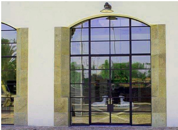
A detailed building entry
