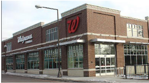
Varied parapet heights and sizes provide interest and variety to this building
